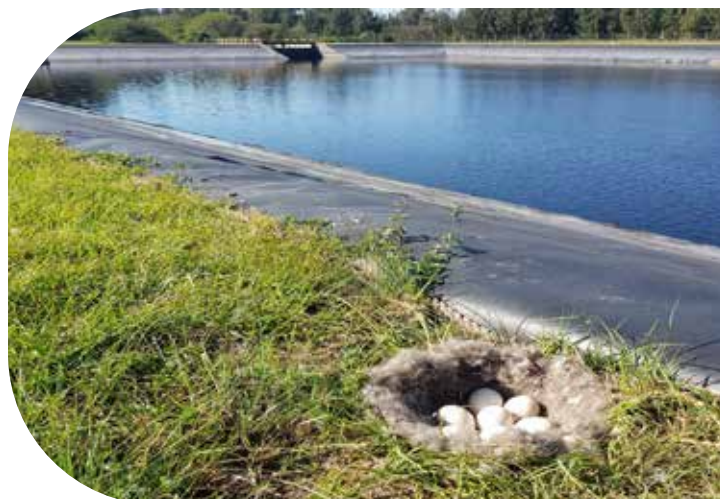
ESUP Dam (Storm Water)
